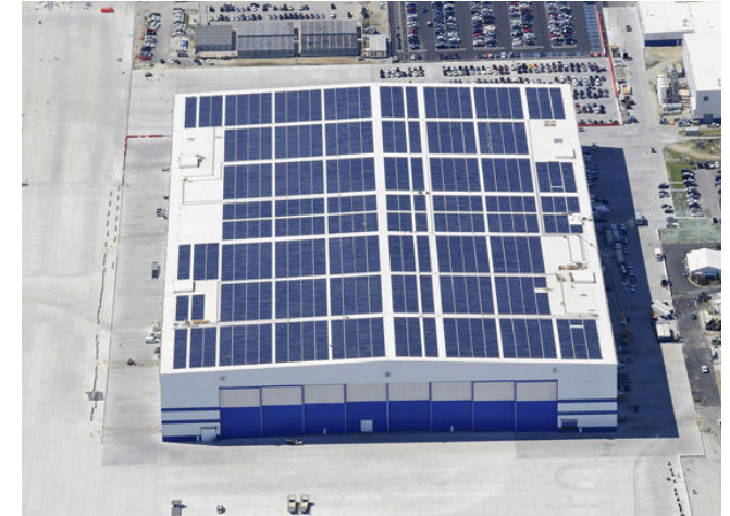
BOEING'S ROOFTOP SOLAR ENERGY FARM, NORTH CHARLESTON, SC
